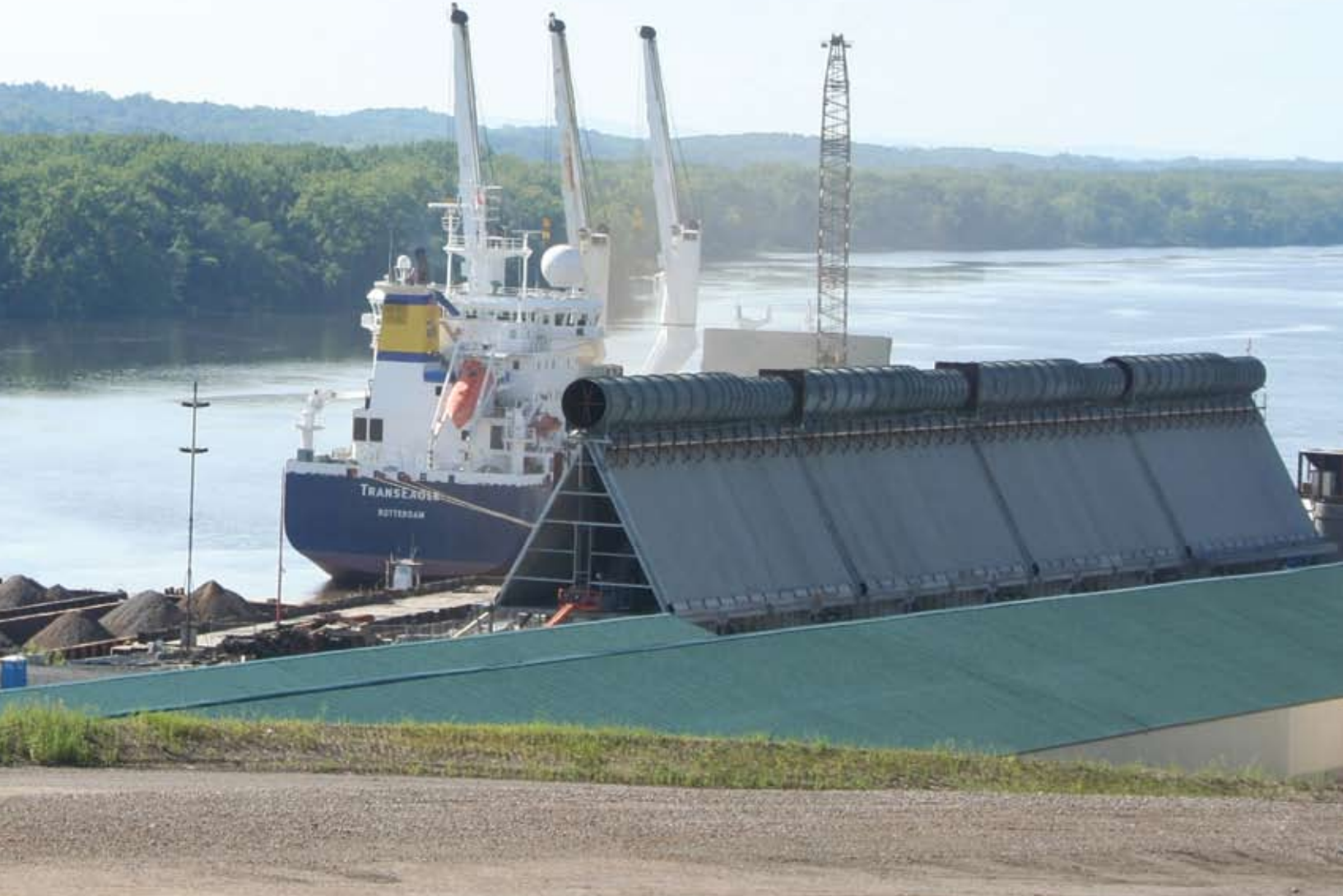
The Port's 115ZV-2 tackles a wide variety of materials including salt, gypsum, slag, bauxite, sand, gravel, and harbor stones. The tent-like structures in the background are actually a part of Migrant Corporation's 24-cell GEA air-cooled condenser for the Astoria II Generating Station in New York City. It is the largest project of its kind to address the power-generation needs of New York.
