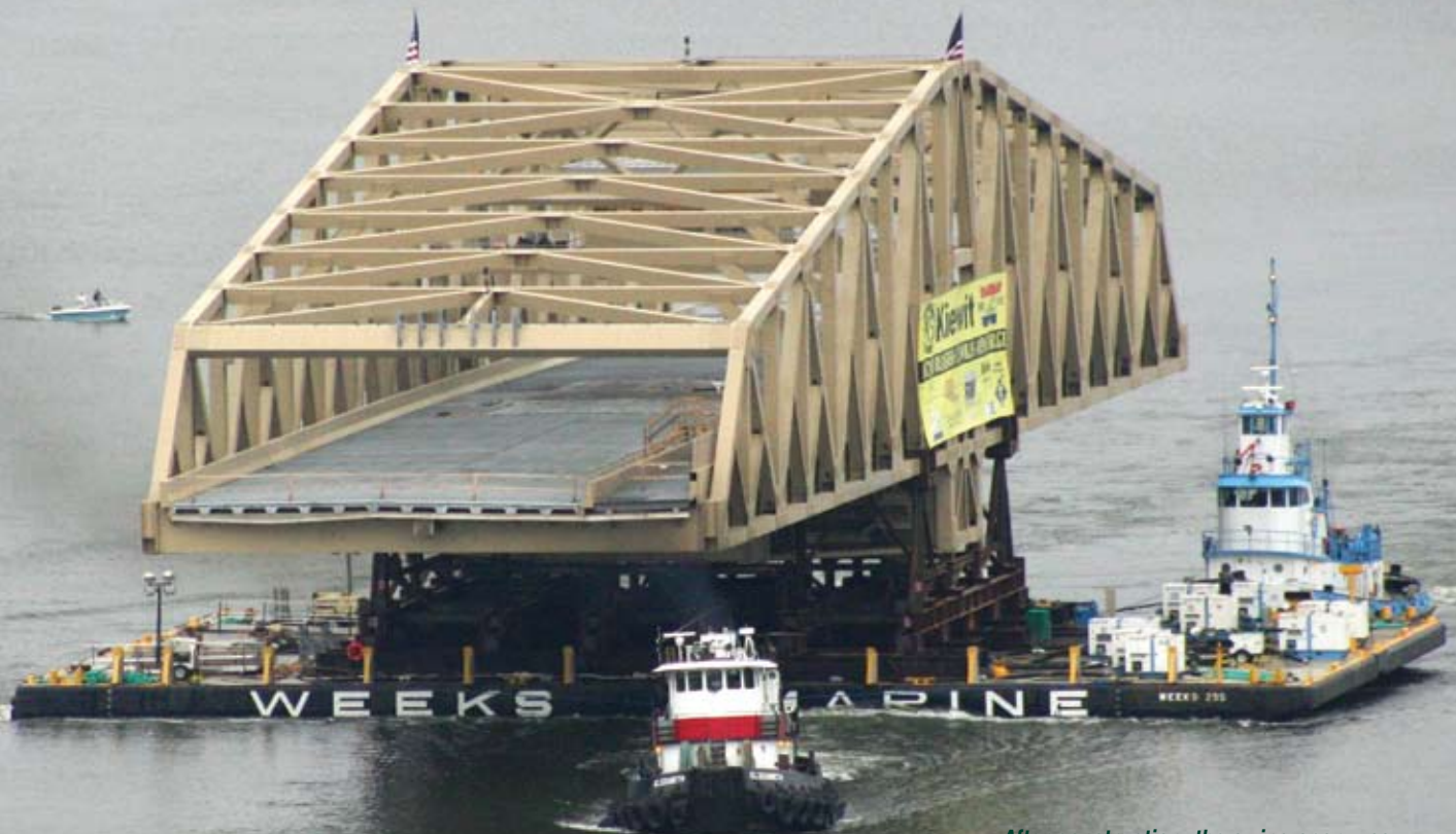
After construction, the swing span was floated down the Hudson on two welded-together barges powered by several tugs.
