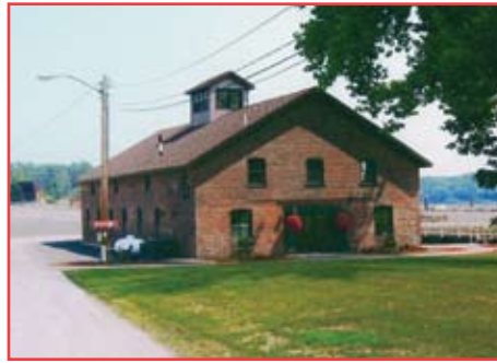
P&M Brick's old horse barn was renovated and now serves as the Port's office.
